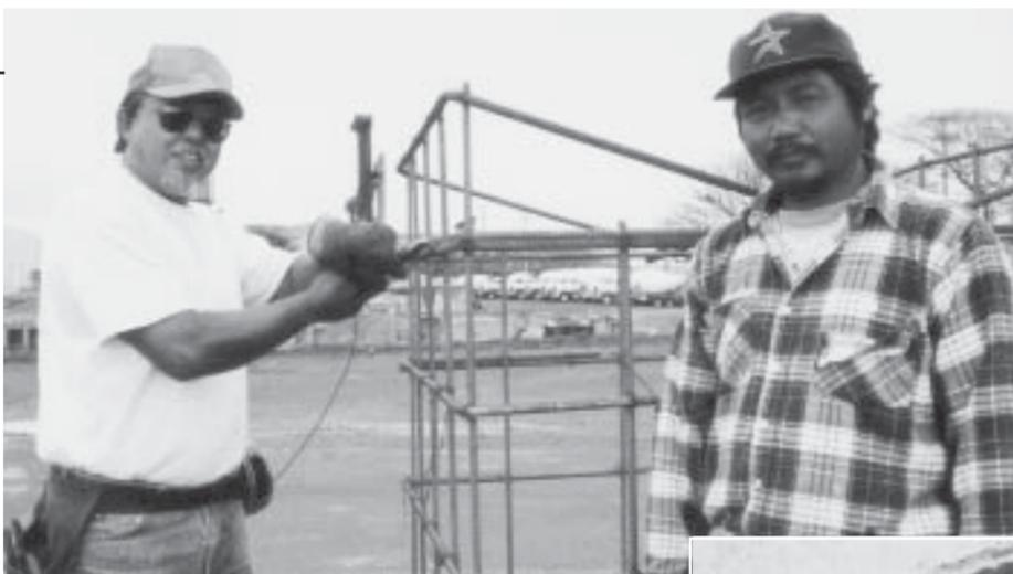
(Left) Steward Sonny Alviar and Laudino Pachico are "pre-cast concrete specialists," shown here fabricating steel skeletons that will be placed into concrete for reinforcement. Alviar became a steward "to be active in the union, and to make sure nobody runs all over us. With the ILWU, the company treats us fair, and we do our fair share—so far so good!"
