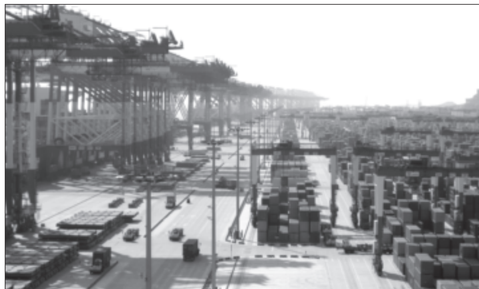
Shanghai, China, is the world's busiest port, handling 29.05 million 20-foot equivalent (TEU) containers. The Yangshan Deep-Water Port in Shanghai (above) was built in 2005. It can handle container ships of up to 8,500 TEU. Photo by Reb42 under a free public license from Creative Commons.
