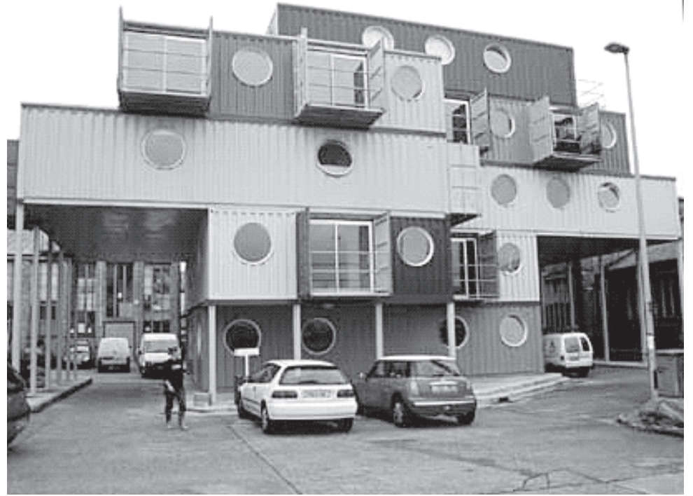
Container City on Trinity Buoy Wharf in London used 45 containers to create 34 studio apartments.
