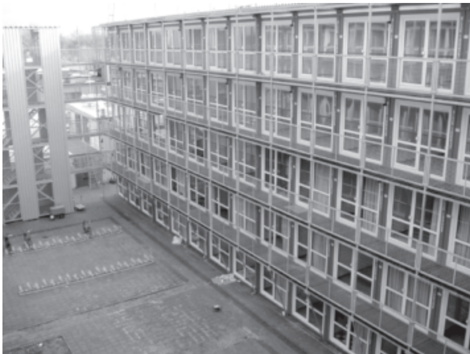
The Keetwonen student housing is made from 1000 containers stacked five-high in the city of Amsterdam, Netherlands.
